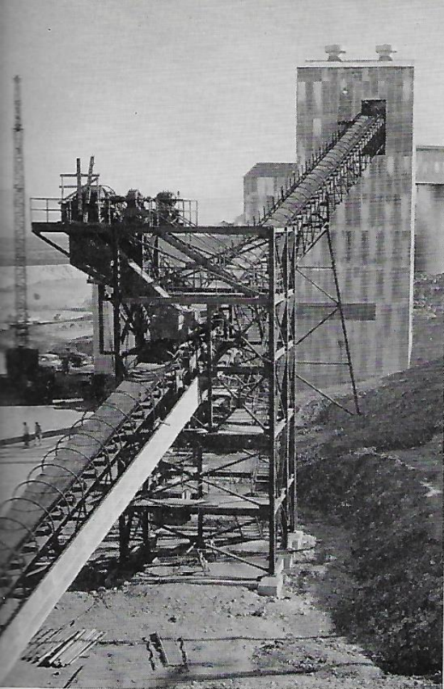
The mill includes primary, secondary and tertiary crushers — rod mills and ball mills — and a flotation unit equal to 200 tons of 25% copper concentrate per day.
