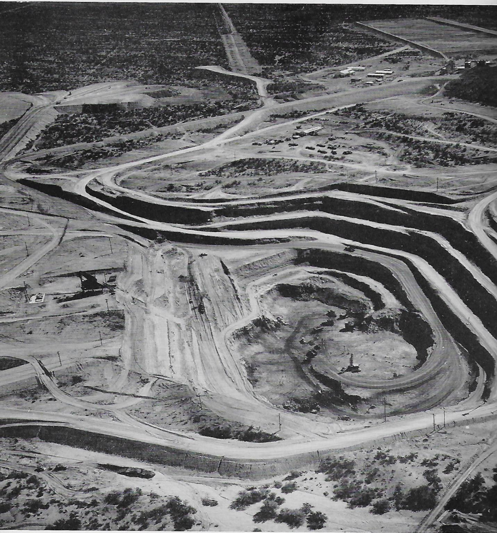
The bottom of Pima Mine's open pit is the top of a valuable ore body discovered through geophysical methods. Walter E. Heinrichs, Jr., left, was one of the prospectors chosen by Herbert Hoover, Jr. Another, Robert E. Thurmond, is introduced on a following page.
